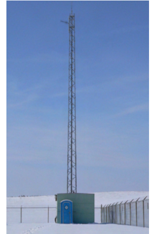
Typical self-supporting telecommunications tower.
