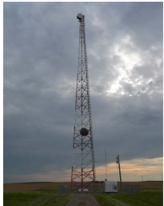
A typical self-supporting telecommunications tower
