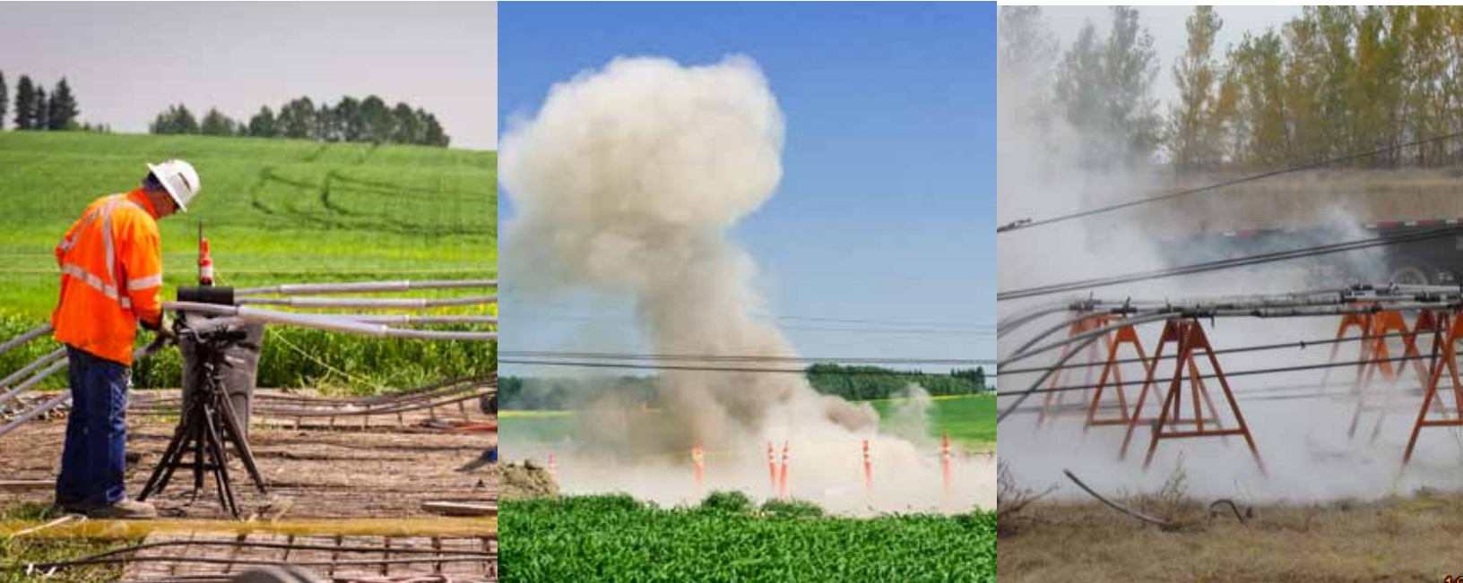
Photos from left to right: wires being prepared for implosion, implosion caused by implosive connectors, wires fused together following implosion.
