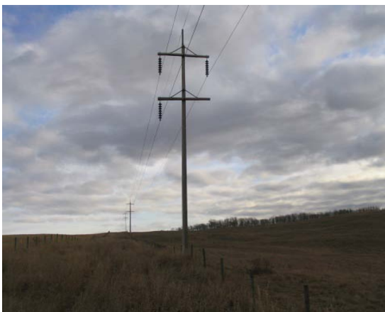
The proposed new transmission structures will look similar to the single-pole structure pictured here. The structures will be made of wood, steel or composite material.
