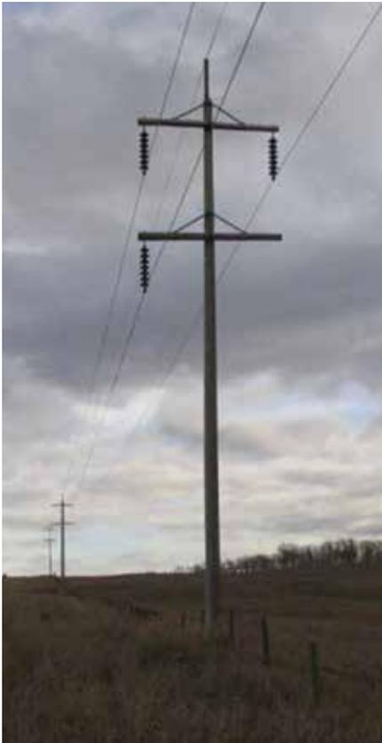
*138 kV single circuit transmission structure*
