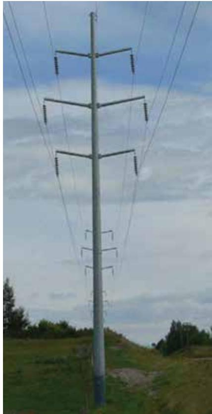
*138 kV double circuit transmission structure*
