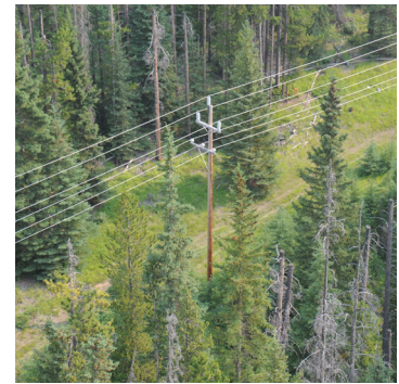
Above: One of the structures that will be replaced as part of this project.
