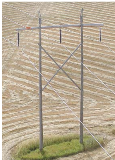
Two pole structure similar to the proposed
