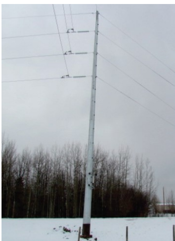
Bottom: the proposed structure will look similar to the structure pictured below.
