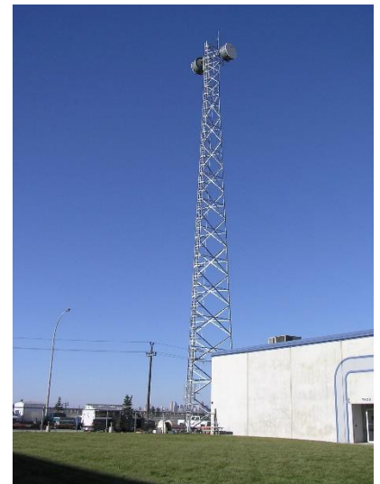
The existing Foothills telecommunications tower
