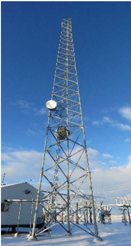
The new telecommunications tower will look similar to the tower in the image above.
