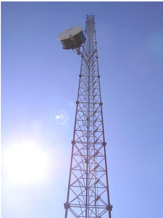
The new telecommunications tower will look similar to the tower in the image above.
