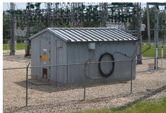
The existing control building
