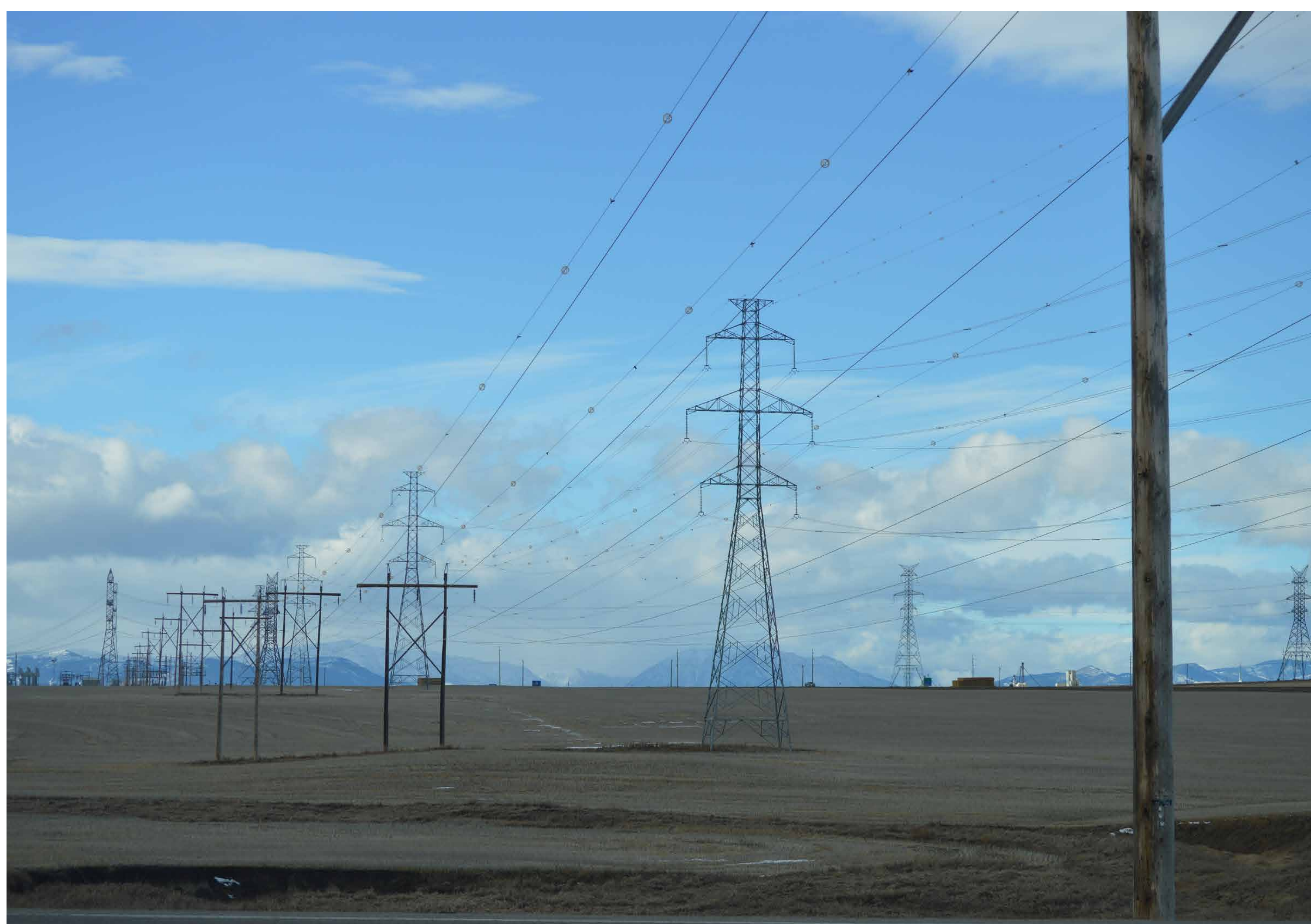
Installed bird diverters
