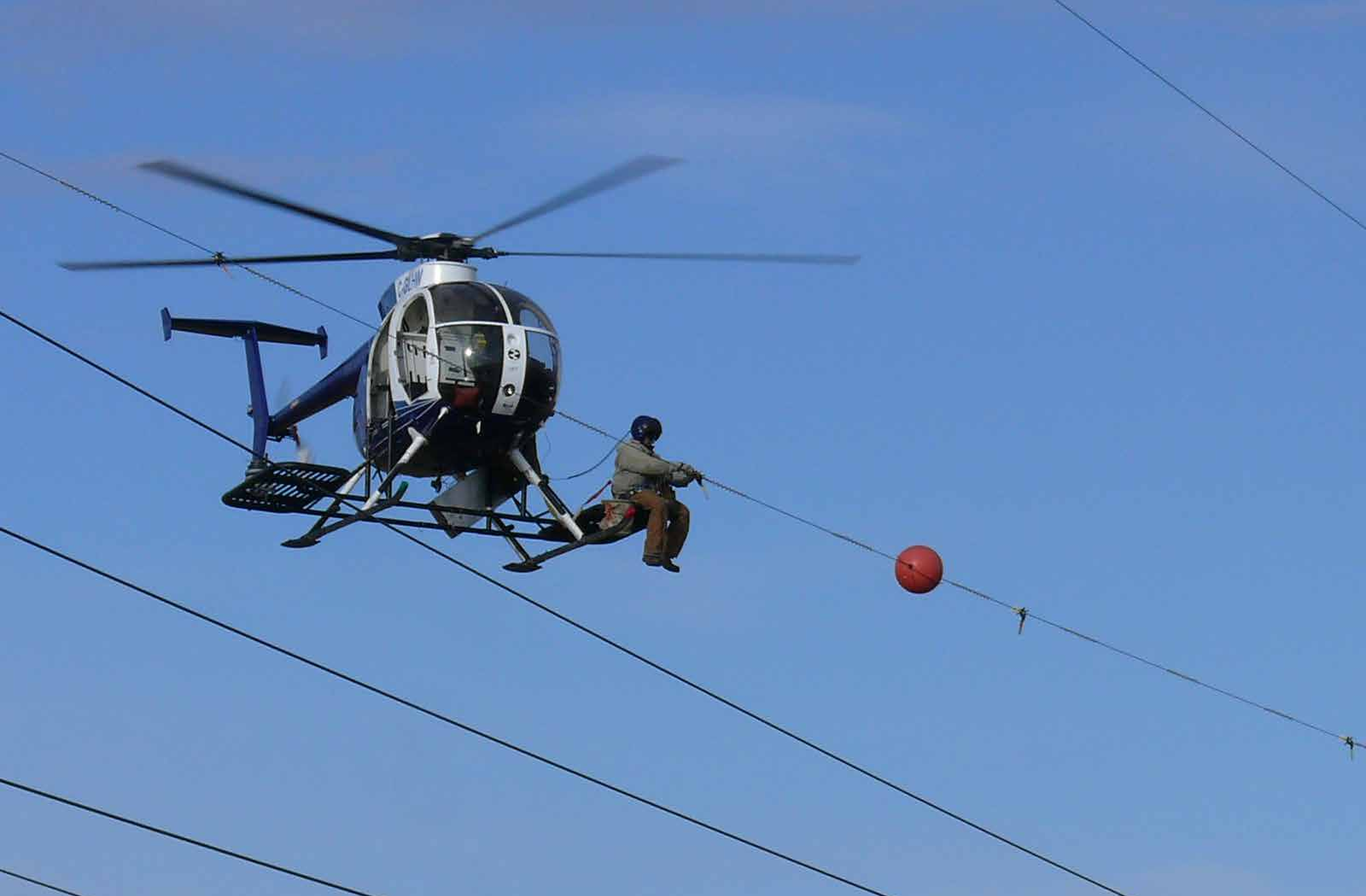
Bird diverter installation
