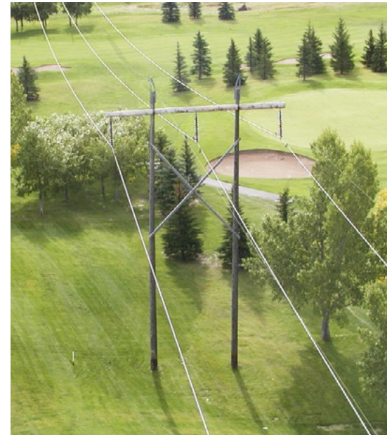
The 150L Transmission Line Rebuild involves rebuilding 30 kilometres of 138-kilovolt transmission.
