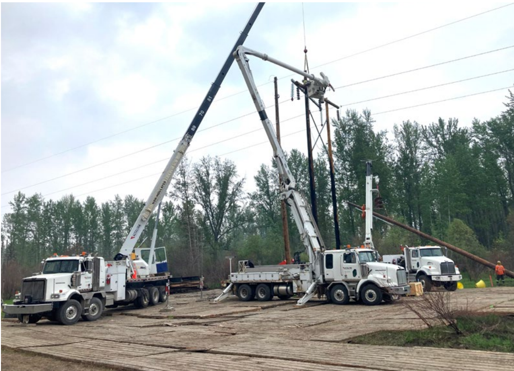
Bottom: Access mats helped crews complete repairs in difficult site conditions.
