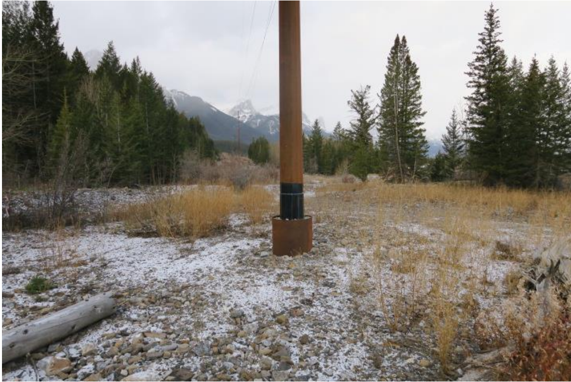
Image of installed screw pile.
