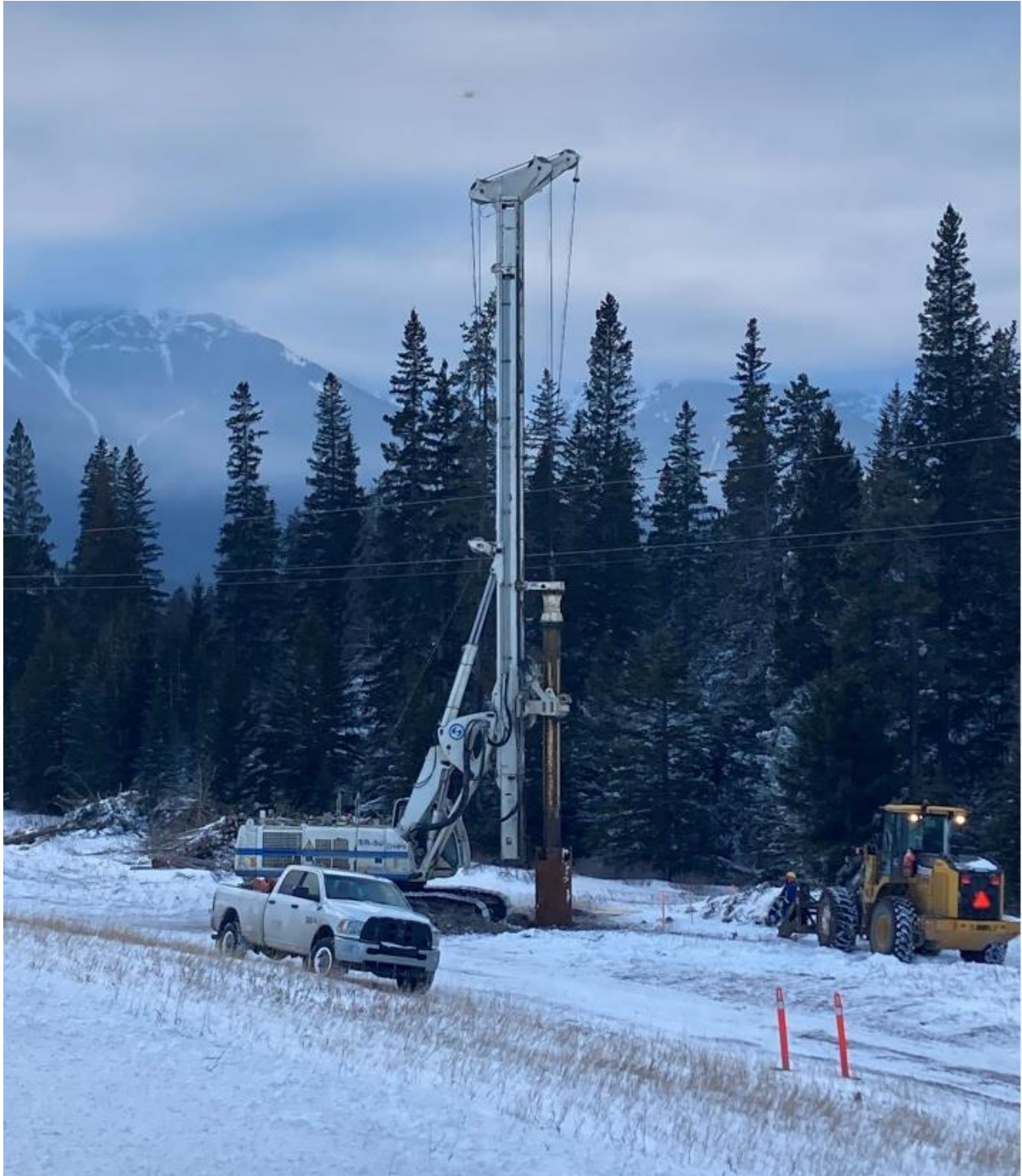
Image of screw piles being installed on an AltaLink transmission line.
