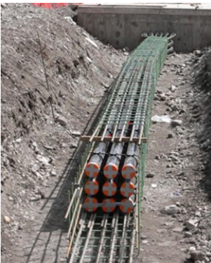
Example of underground conduit for duct being placed in a trench before concrete is poured
