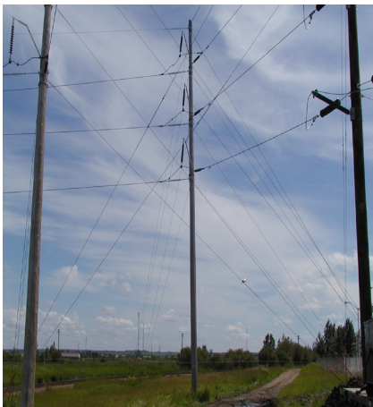
The existing 787L31 structure is shown in the photo above
