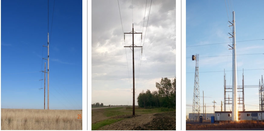
Left: the existing monopole structures on the 853AL transmission line Centre: an example showing the proposed monopole structures Right: an example showing a proposed steel monopole structure
