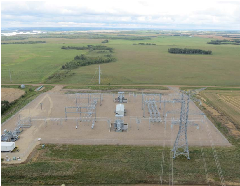
Existing Nilrem Substation
