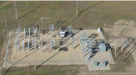
Existing Edgerton Substation
