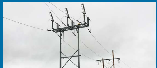
A typical airbreak
