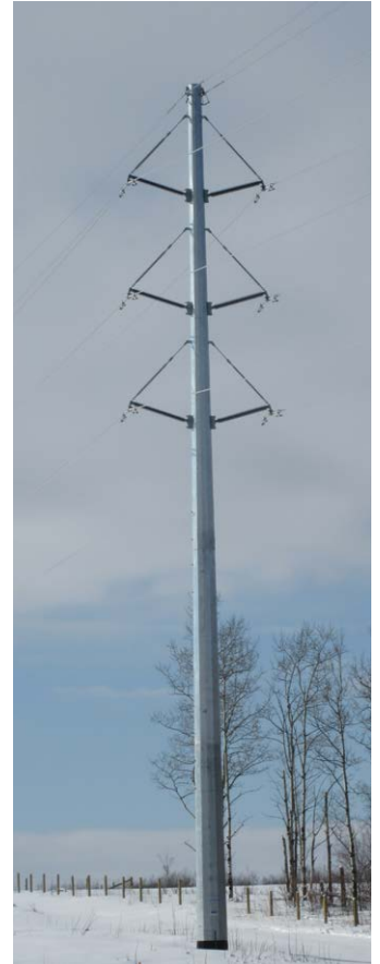
The double circuit 240/69 kV structures will look similar to the structure pictured here.
