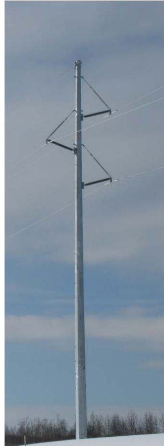
The 69 kV structures will look similar to the structure pictured here.
