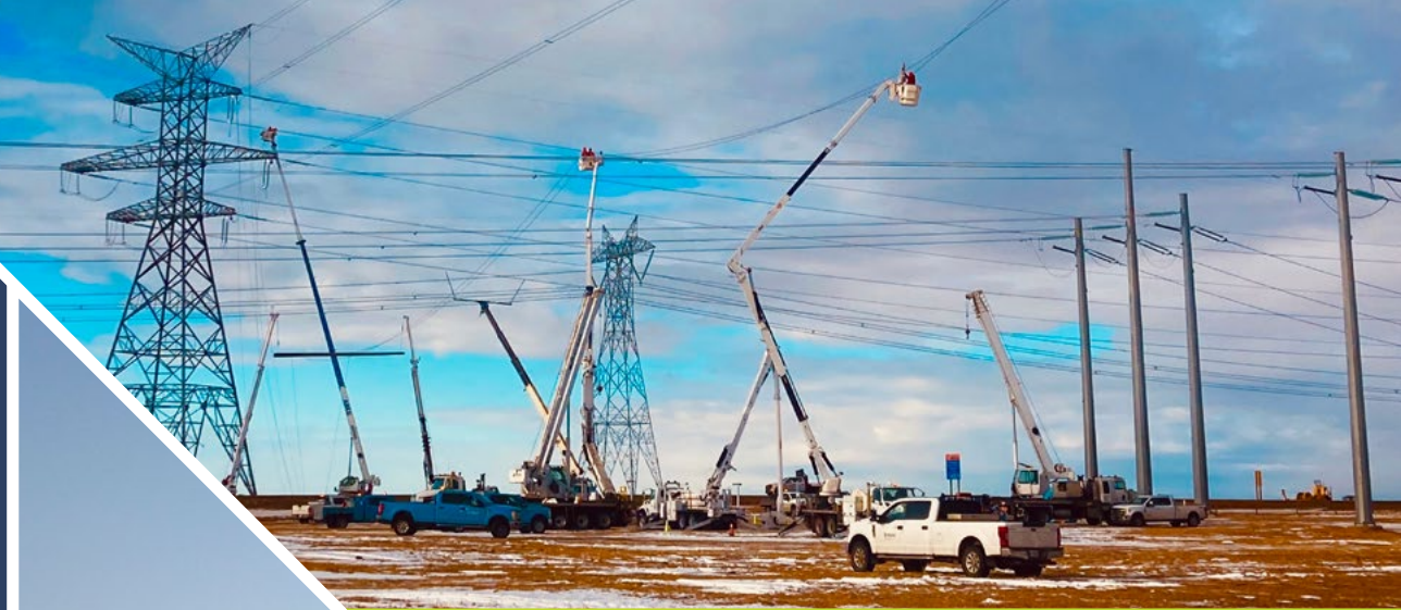
▲ Teams working to restore transmission lines following the Brooks storm
