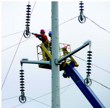
Above: Once structures are erected, transmission line wire, called conductor, can be strung.
