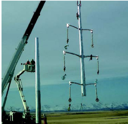
Above: AltaLink will assemble and erect steel pole structures.
