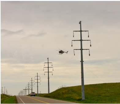
Above: Residents may see a helicopter in your area performing conductor (wire) stringing and hanging markers and hardware along the CETO transmission line
