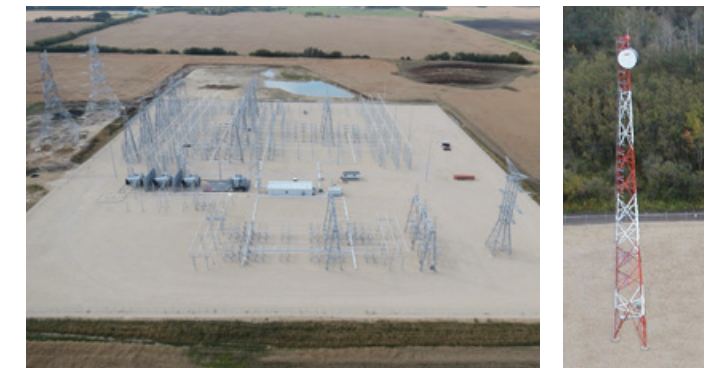
The Chapel Rock Substation will look similar to the one pictured here. Telecom tower.
