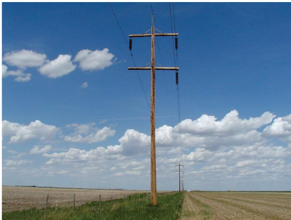
The existing 831L line near the proposed project area.
