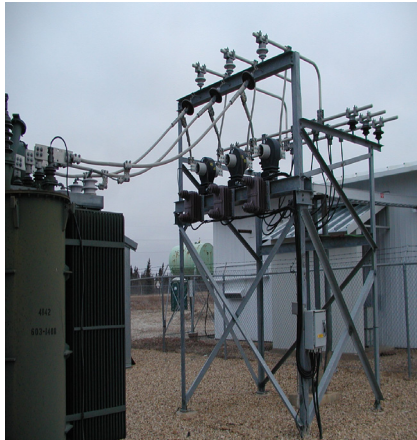
The existing transformer being removed is in the photo above
