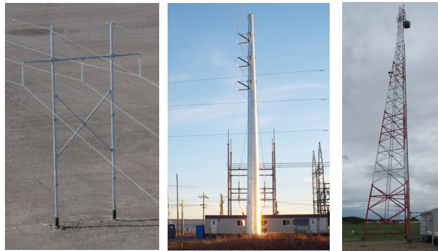
Left photo: The proposed H-Frame structures.
