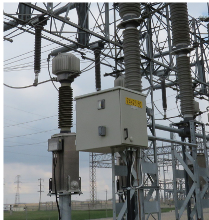
The existing circuit switcher is pictured to the left. The new circuit breaker will look similar to the picture on the right.
