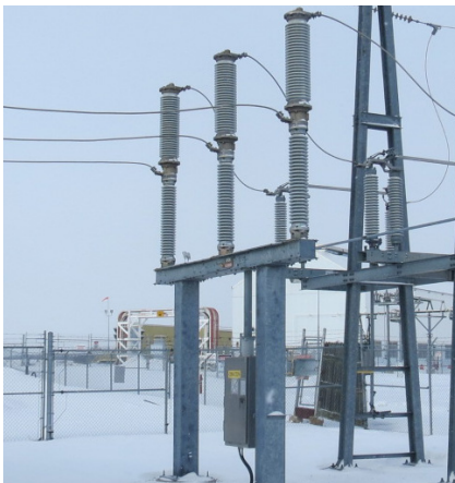
The existing circuit switcher is pictured to the left. The new circuit breaker will look similar to the picture on the right.
