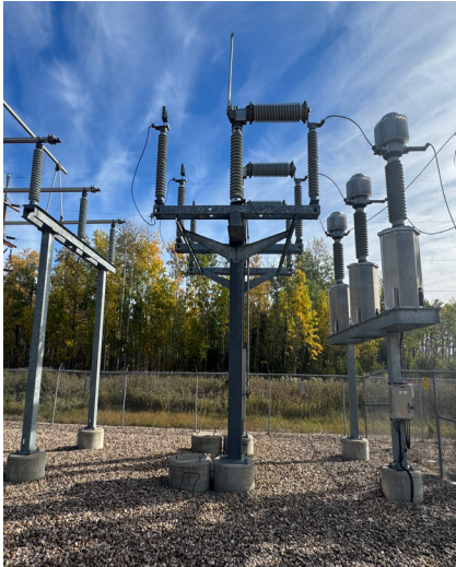
The existing circuit switcher is on the left. The new circuit breaker will look similar to the picture on right.
