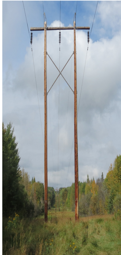
Above: Wood H-frame structures will look similar to the one shown in the photo
