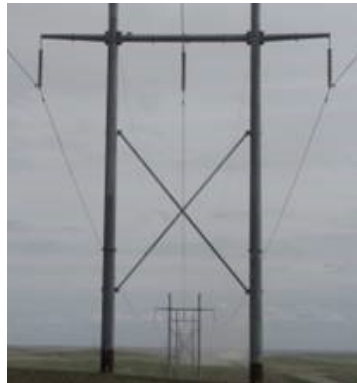
The proposed structures will look similar to the H-frame structure shown above and may be wood or steel.
