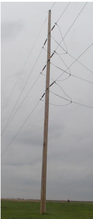
The new structure will look similar to the photo above.
