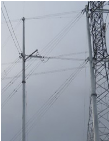
Top: an example of a single pole structure
