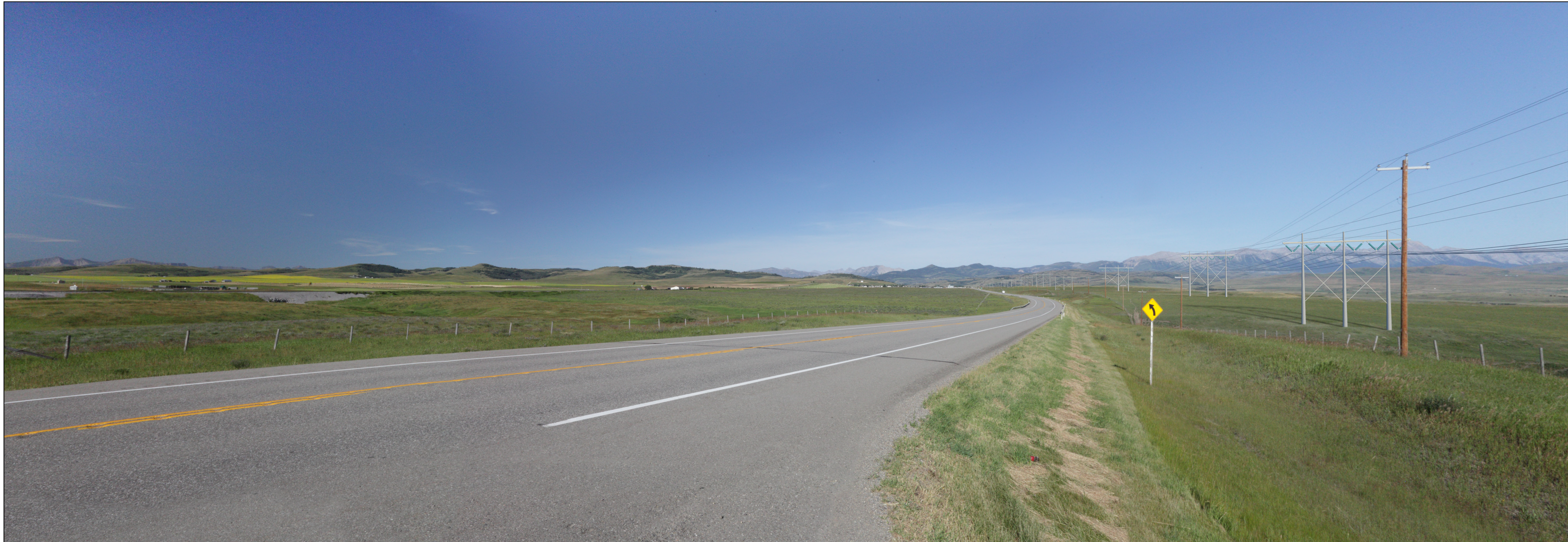
Viewpoint SH1 - Highway 3 (Crowsnest Highway - East of Lundbreck), Looking West-Southwest - Structure 5
