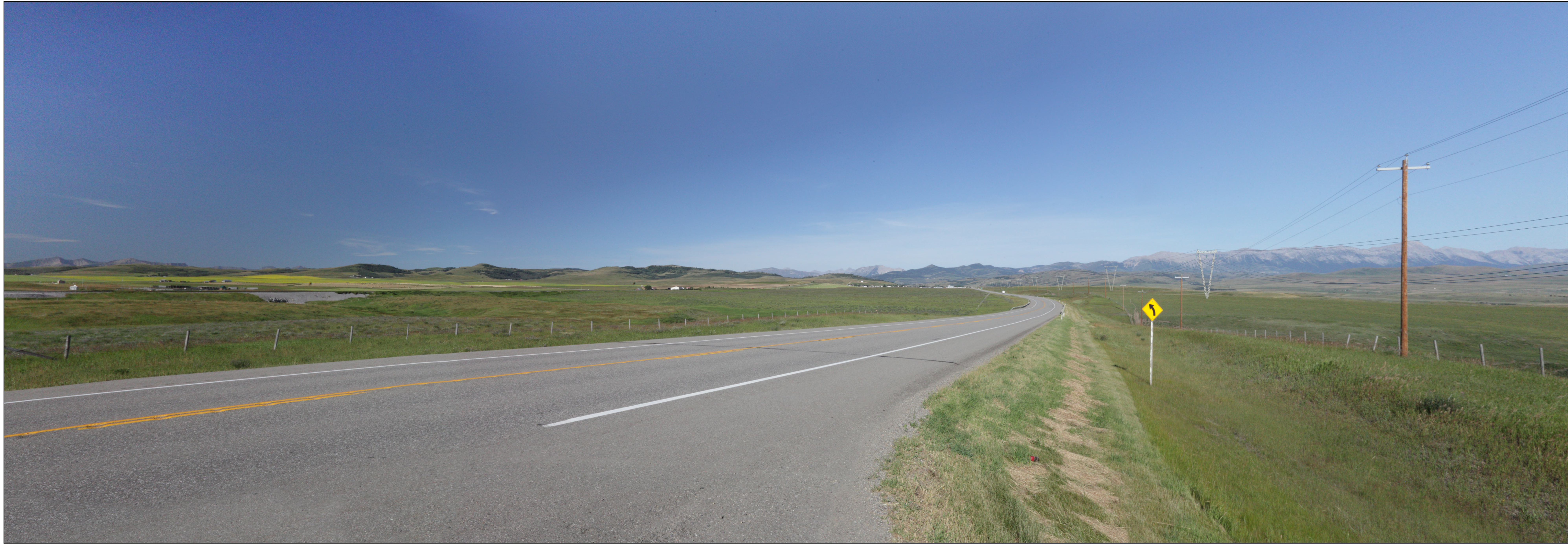
Viewpoint SH1 - Highway 3 (Crowsnest Highway - East of Lundbreck), Looking West-Southwest - Structure 1
