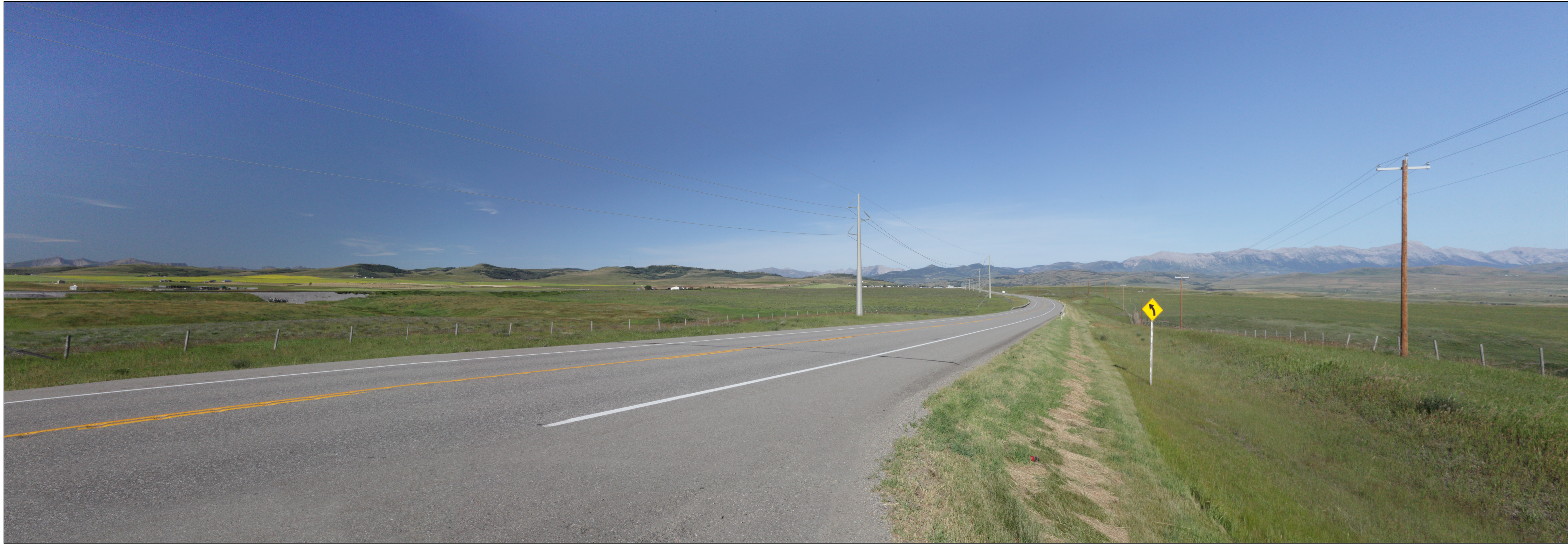
Viewpoint SH1 - Highway 3 (Crowsnest Highway - East of Lundbreck), Looking West-Southwest - Structure 3
