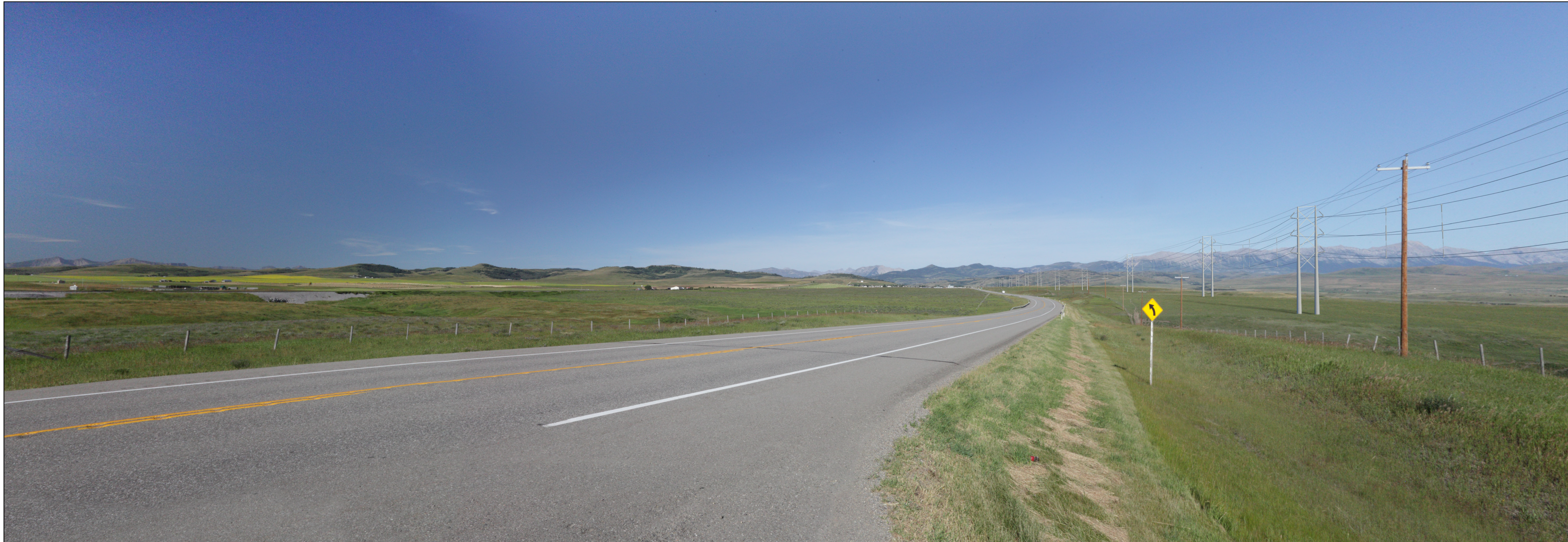
Viewpoint SH1 - Highway 3 (Crowsnest Highway - East of Lundbreck), Looking West-Southwest - Structure 7
