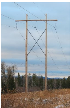
The image on the left is an example of the existing H-frame structures and the image on the right is an example of what the replacement H-frame structures and hardware replacements will look like.
