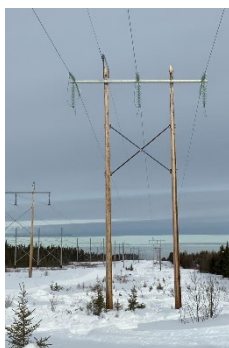
The image on the left is an example of the existing H-frame structures and the image on the right is an example of what the replacement H-frame structures and hardware replacements will look like.
